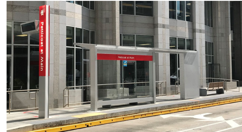
Level-boarding Curb with Rub Rail (MAX – Kansas City, MO)
