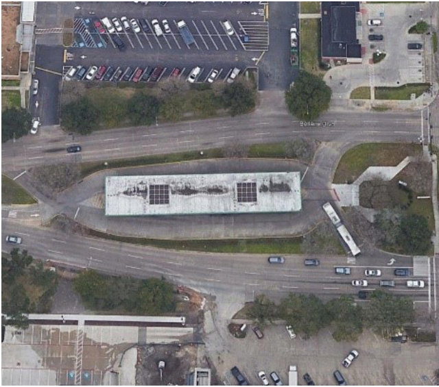
FIGURE 5-8: BELLAIRE TRANSIT CENTER, HOUSTON
