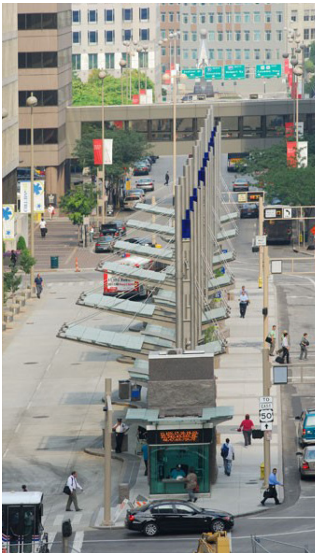
FIGURE 5-6: GOVERNMENT SQUARE TRANSIT CENTER, CINCINNATI
