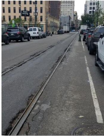
Deteriorating Asphalt Along St. Charles Streetcar Line
