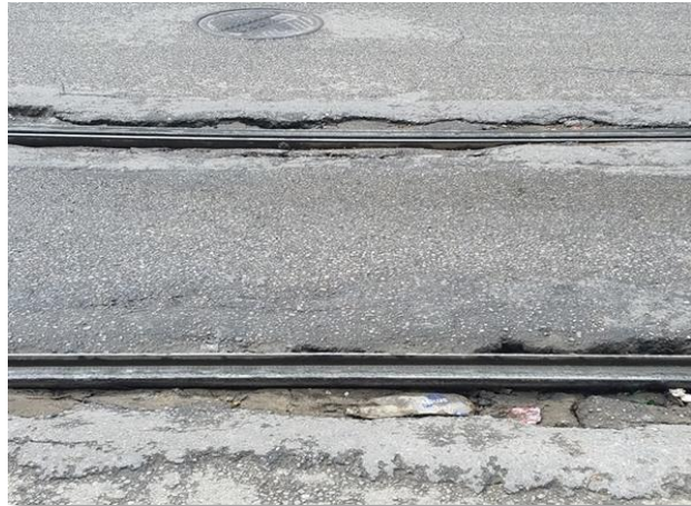
Deteriorating Asphalt Along St. Charles Streetcar Line
