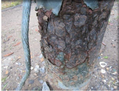
Corrosion on base of poles
